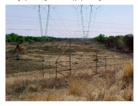
**Figure 3.** A game fence as used on the Matimba-Spitskop 1&2 lines. Note that the top section has been omitted as per the latest 5m game gate design.
